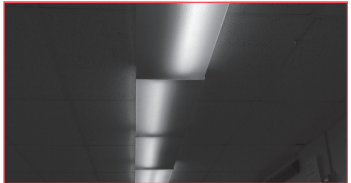
Lighting fixtures throughout the building need to be replaced
