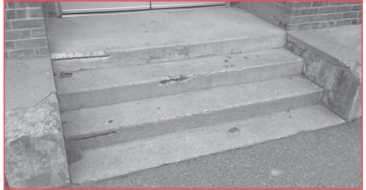
Masonry work is needed on steps, sidewalks, and other areas
