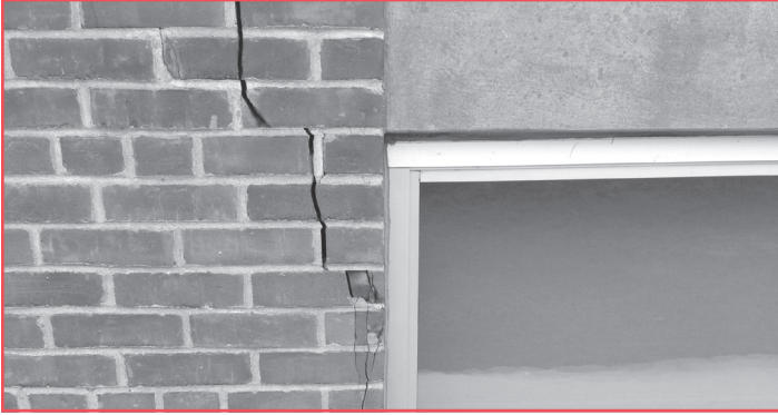
Cracks throughout the main building's foundation need repair
